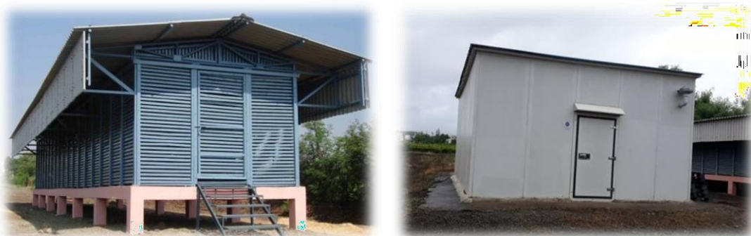
(a) Bottom and side ventilated double row structure, (b) Controlled Onion Storage Structure Fig. 7. Onion storage structures developed by ICAR-DOGR
