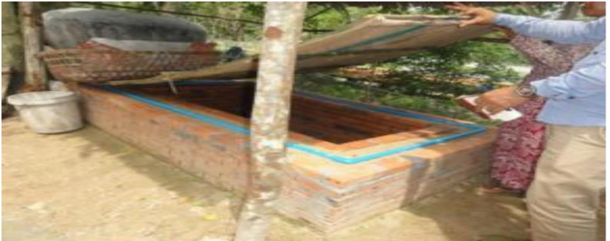
Fig 1: Zero Energy Cool Chamber for highly perishable fresh horticultural produce
