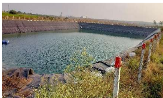
Creation of water facility for irrigation
